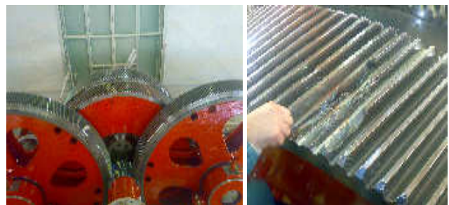
Figure 5. Disassembling of the reducer and damaged wheel
