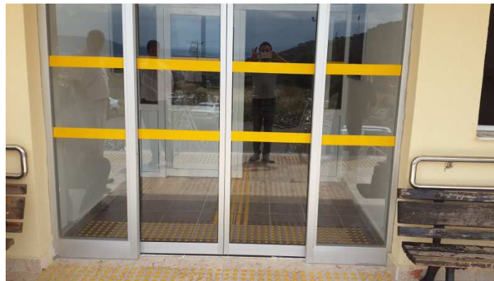
Fig. 8. An example of applying warning tapes on glass surfaces, Yalova Armutlu state hospital (Archive of Sahin Durak, 2016)
