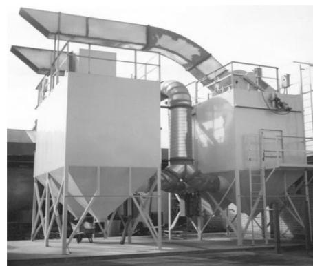
Figure 2. A twin-module baghouse of the zinc galvanizing facility
