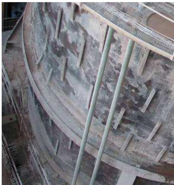
Figure 2. The damaged wall of the air conditioning tower between the fixation rings and above them
