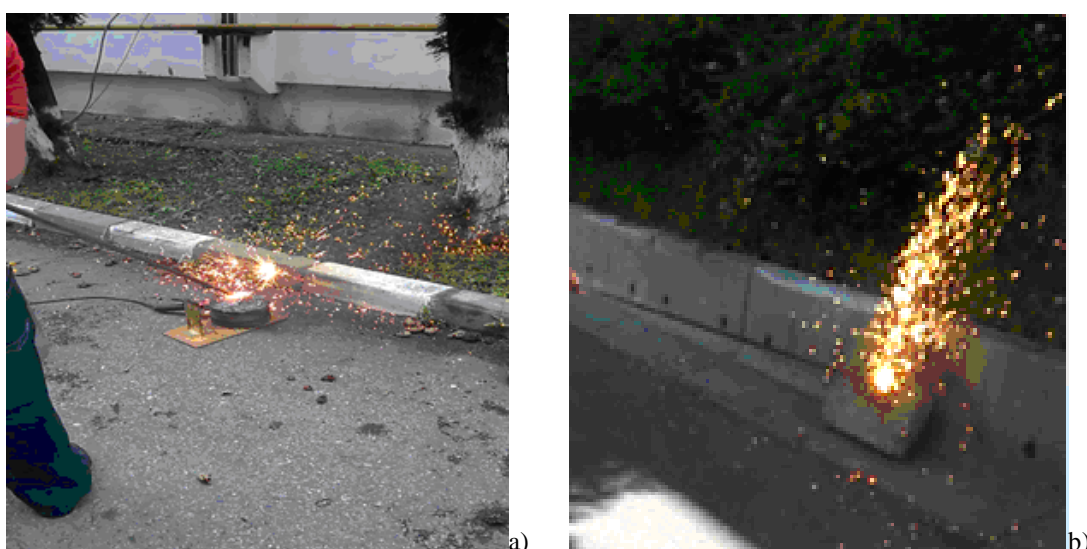
Figure 8. Thermal lance cutting
