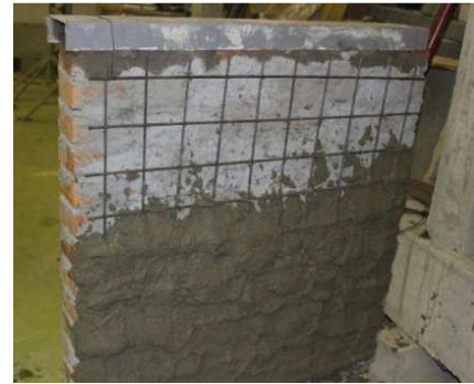
Fig. 4. Strengthening wall with layer of mortar
