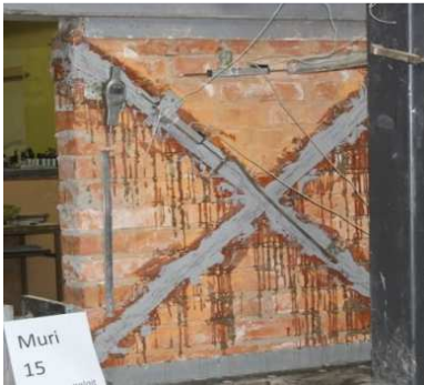
Fig. 3. Strengthening wall with GFRP
