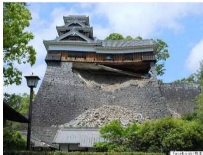
Fig. 2. Foundation stones collapsed [11]
