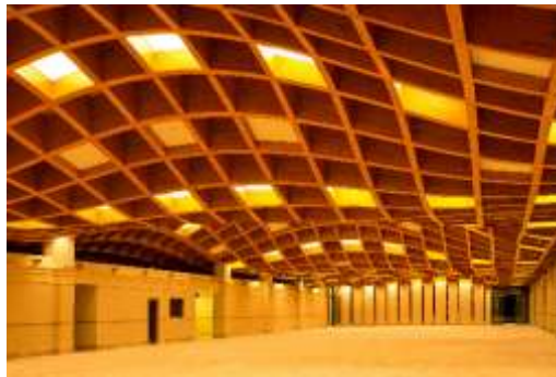
Fig. 1. Glulam system. Openings of 108 metres. Avcılar Nikah Salonu (Naswood Archive)
