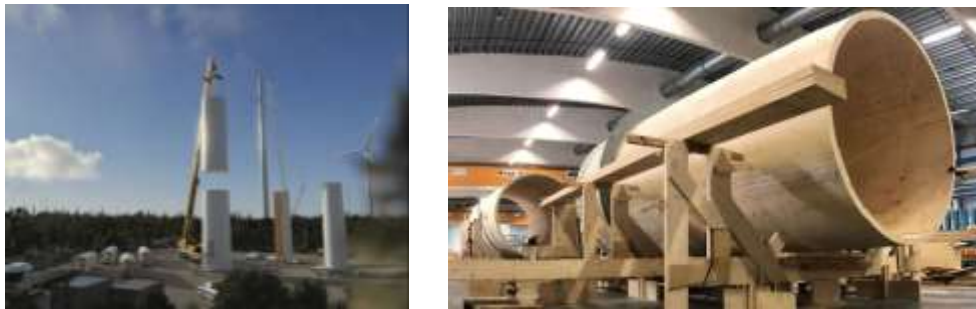
Fig. 4. Wooden Wind Turbine built with LVL Height 105 m. Sweden (Modvion Archive)
